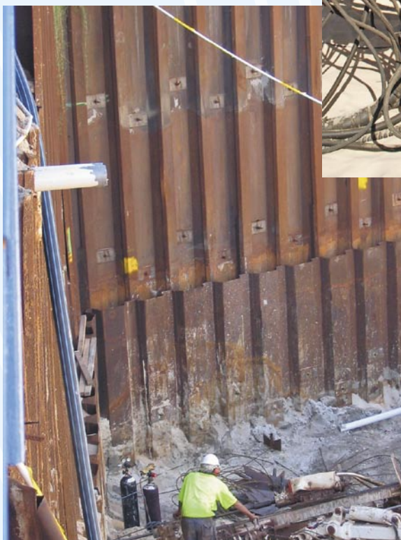
Above: ASP anchoring rig at work.
