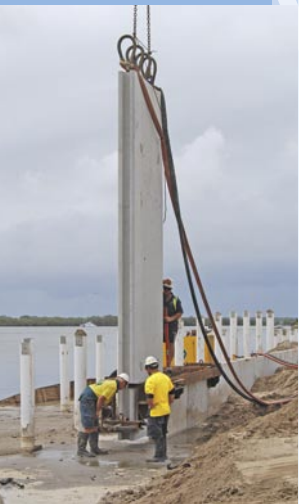
Below: Showing pre-cast panels being jetted into place.
