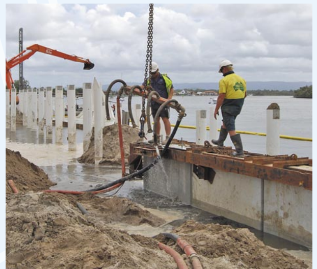
Above: Removing the jet rig and lifting tackle.
