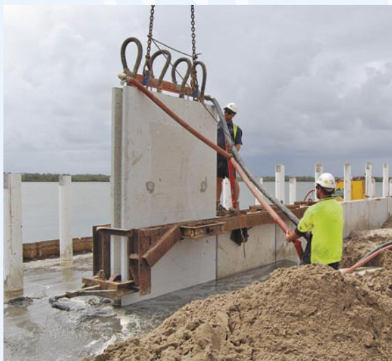
Above: Jetting the panel into position.
