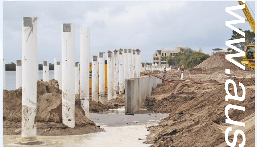
Above: First in this sequence of photographs from the Little Beach Project at Paradise Point, Queensland, we see the partially completed revetment wall with dewatering taking place between the wall and the temporary line of sheet piling. The top edge of the wall is finished with capping beams.
