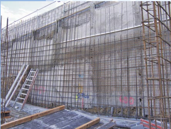
Above: Steel reinforcing used prior to applying a finished spray wall.
