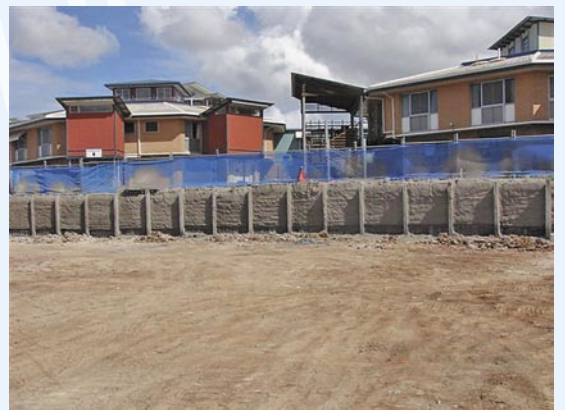
Right: Soldier pile wall faced with shotcrete.
